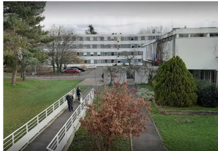
Figure 1 hôpital René Muret APHP
